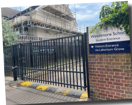
Highfield Road Gate
